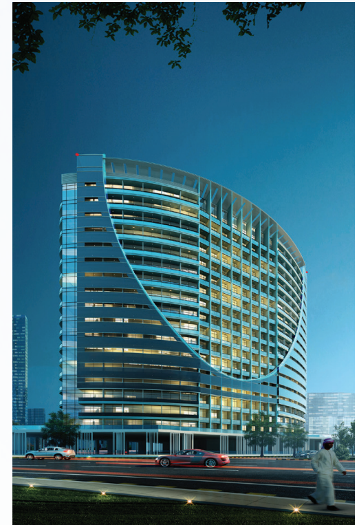
The V Tower
